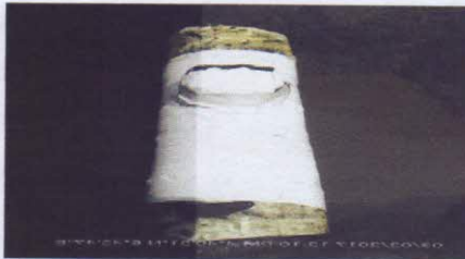
Repaired point with rappers.
