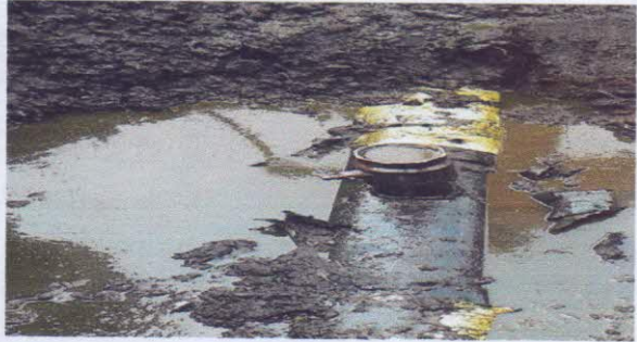
After excavation showing installed valve.
