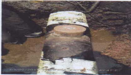
Cone during repair.
